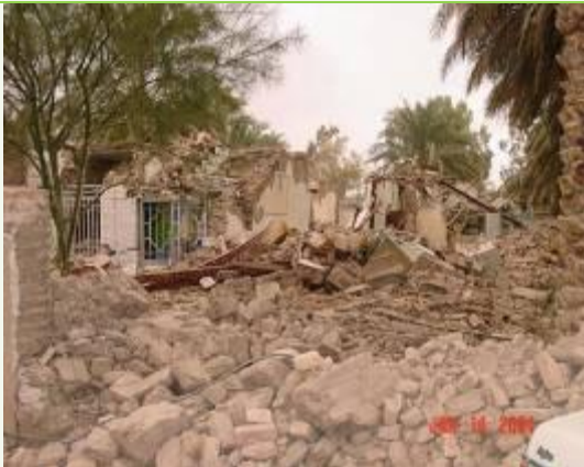
(Source: http://www.worldhousing.net/wherereport1view.php?ID=100130 ) Figure 2-3 Collapsed adobe structures 2003 Bam Earthquake
