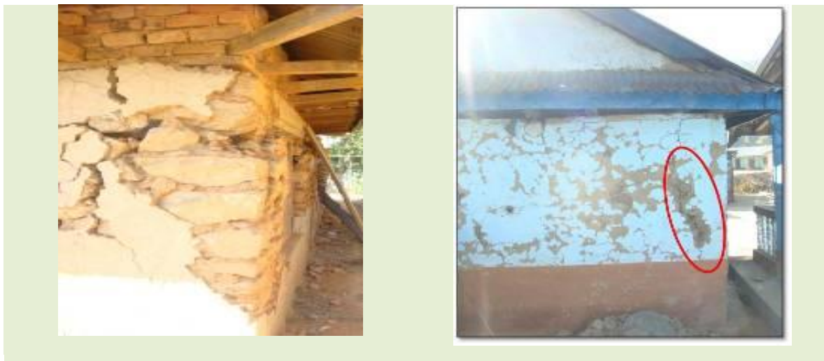
Figure 2-18 Some other examples of corner damages (Source: CoRD)
