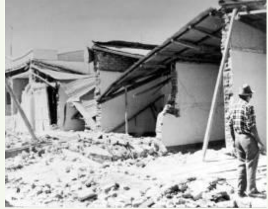
(Source: irapl.altervista.org , figure 69-B, U.S. Geological Survey Professional paper 1002) Figure 2-2 Damage of adobe houses in Guatemala City during Guatemala Earthquake 1976
