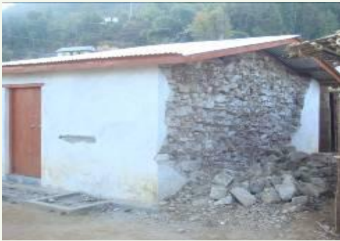
Figure 2-11 Some other examples of Gable wall damage during Eastern Nepal Earthquake, 2011 (Photo: CoRD)
