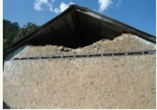
Figure 2-10 Gable end wall mid-height collapse (Sinam, Eastern Nepal Earthquake, September 1st, 2011)
