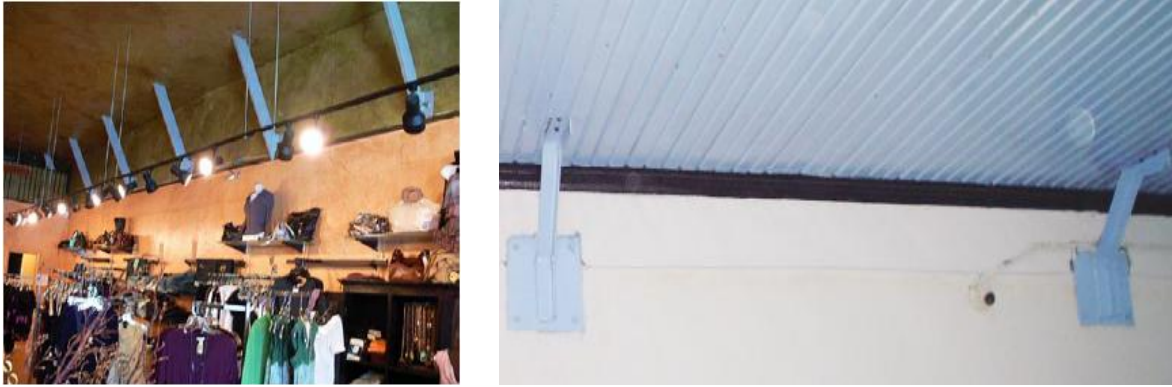
Figure 4-31 Roof to wall connection
