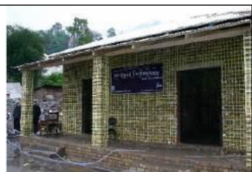
Figure 4-16 PP band retrofitted house before mortar laying (source: Megura and Mayorca)
