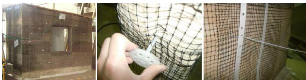
Figure 4-24 Reinforced house with geomesh (Source: world housing tutorial)
