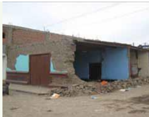
(photo: M. Blondet) Figure 2-8 Out-of-plane wall collapse after the 2007 Pisco, Peru earthquake
