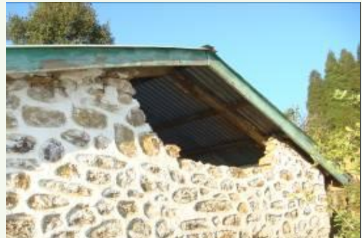
Figure 2-11 Some other examples of Gable wall damage during Eastern Nepal Earthquake, 2011 (Photo: CoRD)
