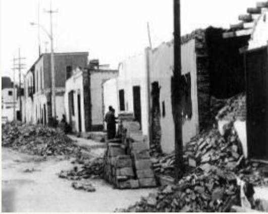
(Source: www.earthquake.usgs.gov ) Figure 2-1 Severe damage to adobe buildings in Chorrillos district in Peru earthquake 1974
