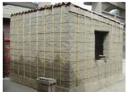
Figure 4-21cane reinforcement
