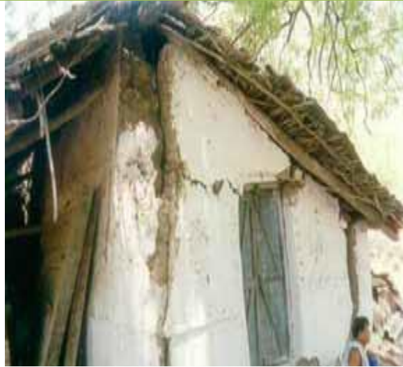
Figure 2-19 Vertical cracking and separation of adobe walls after the 1997 Jabalpur, India earthquake (source: Kumar 2002)
