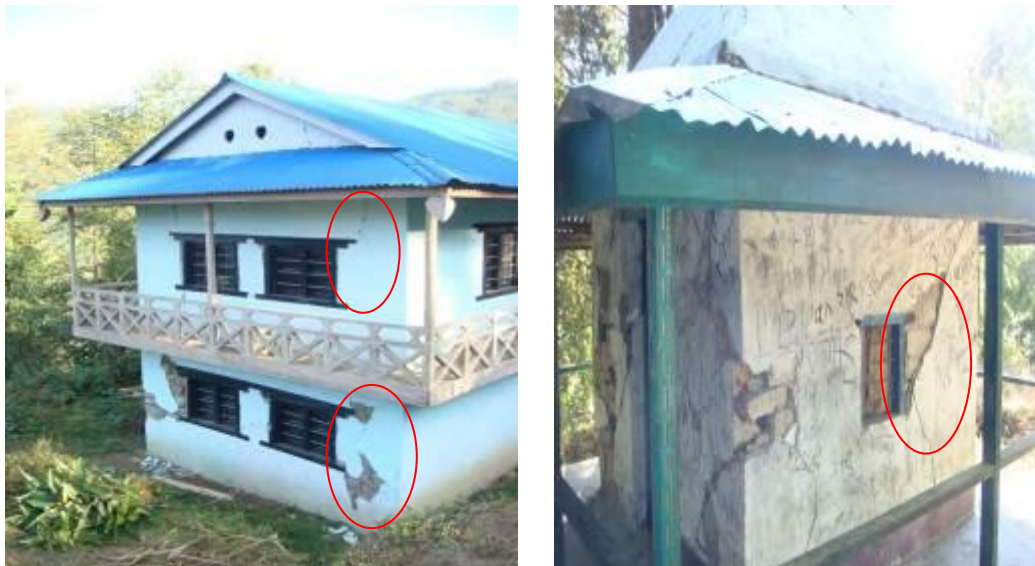
Figure 2-24 Some examples of Cracks at opening (source: CoRD)
