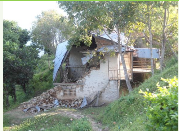
Figure 2-4 Collapsed structure (source: CoRD)
