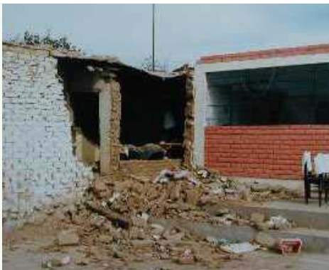
(Source: Report #52 in EERI/ IAEE World Housing Encyclopedia) Figure 2-7 Out-of-plane wall collapse – 1996 Nazca earthquake, Peru
